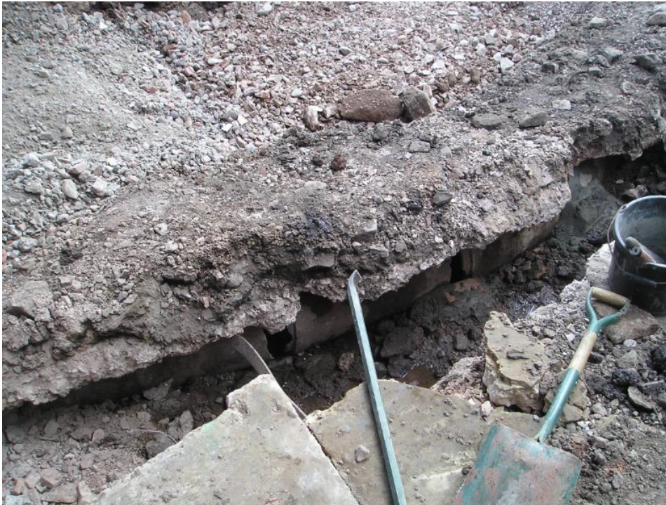
Figure 4-1 – Existing pipe of approximately 450mm in diameter
